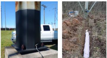
✓ Application of coatings below-grade is the primary method of protection for the majority of buried steel structures
