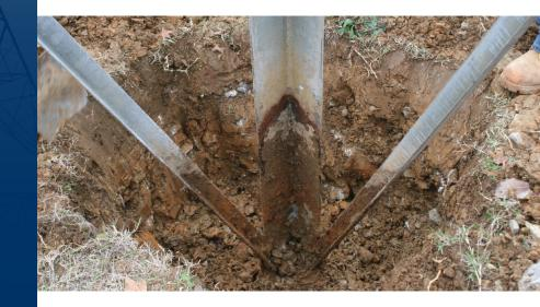
In the U.S., the average age of a steel tower in service is more than 60 years old. Clearly, steel transmission structures are now showing their age.
