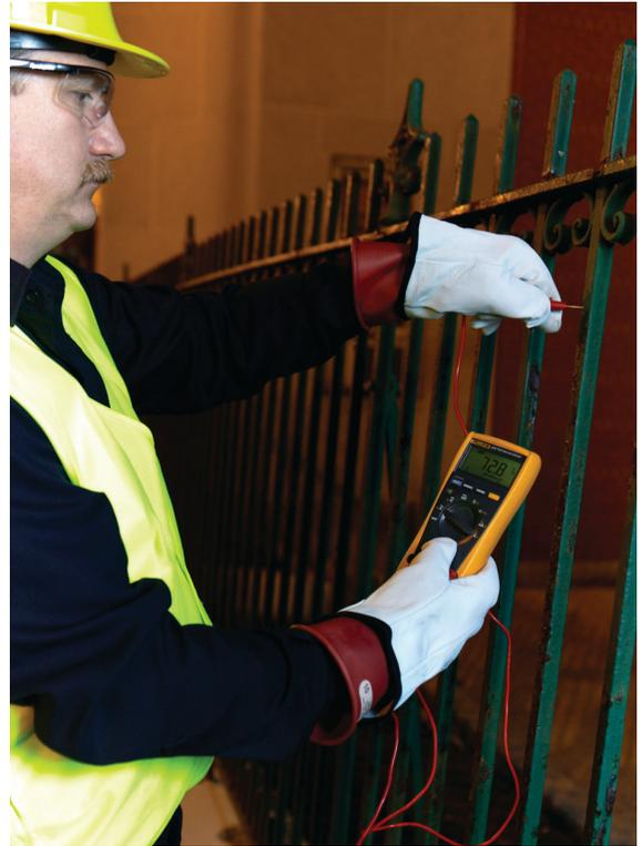
A technician checks a steel fence for contact voltage using a voltmeter and a shunt resistor.
